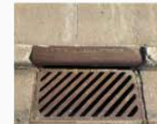
Figure 20 - Storm Sewer Intake
